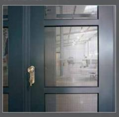
Doors with perforated steel sheets to ensure necessary air circulation.
